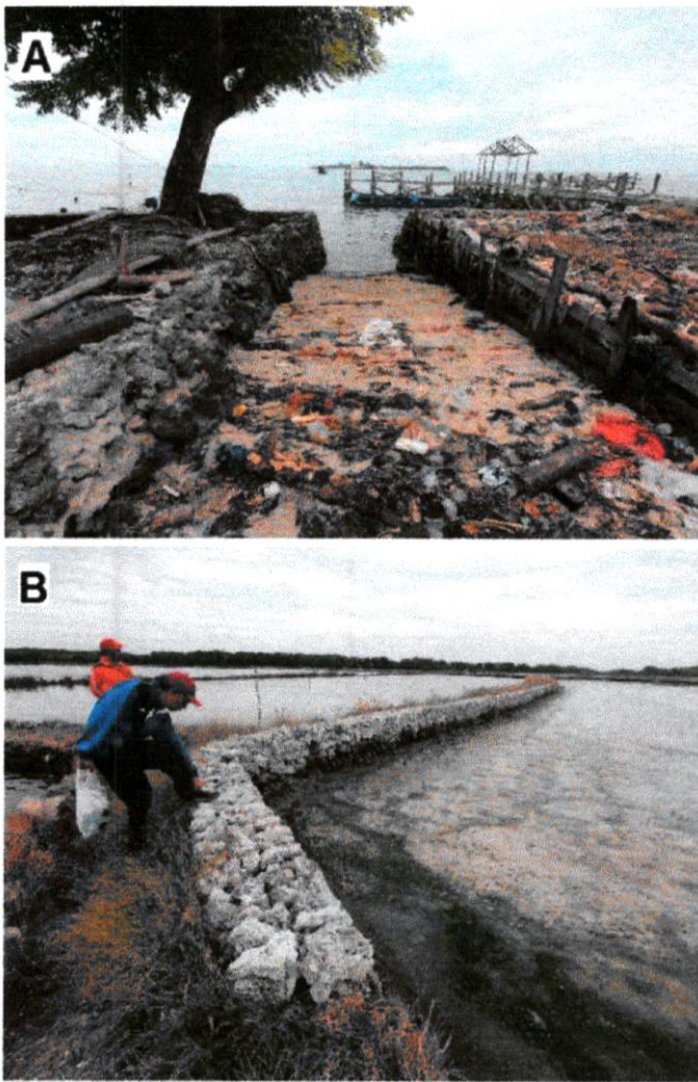
Fig. 2. A. Coral rubble employed to reinforce coastal walls, and B. Dead corals employed to build walls of aquaculture ponds. Both photographs taken by Sarah Hamylton at Sabangko Island, July 2019.
