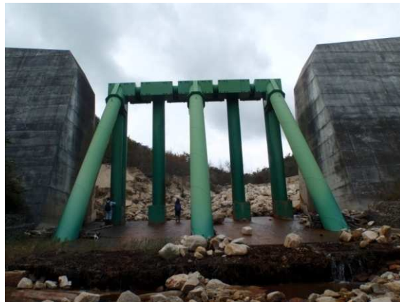
Gambar 5. Cek dam pipa baja di Sungai Hachimandani
