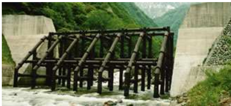
Gambar 4. Cek dam tipe grid pada Sungai Ikazawa Propinsi Niigata Japan (Source: Sustainability Report-Kobe Steel Group Sites, 2011)
