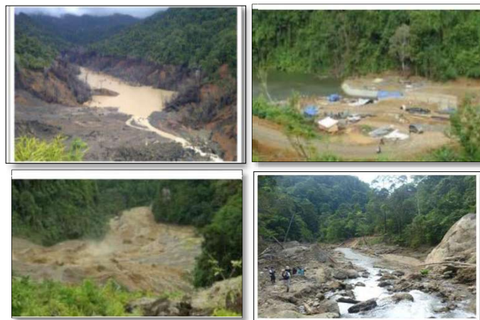
Figure 4. Debris flow Condition post crumbling natural dam.
