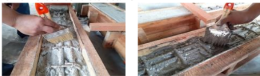
a) Normal concrete surface cleaning b) Bonding agent application
